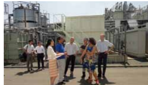
Visit to Hiagari Sewage Treatment Plant
