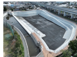
Construction of retention ponds for flood and inundation control
