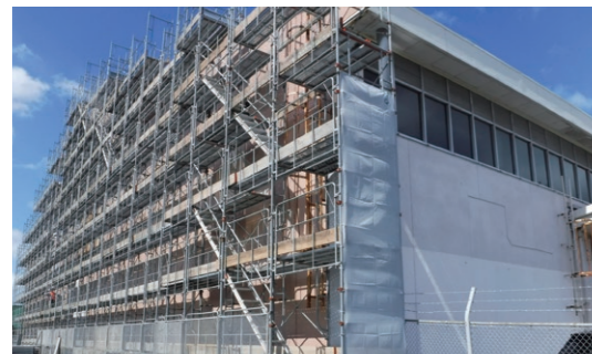
Renovations to extend the service life of public facilities
